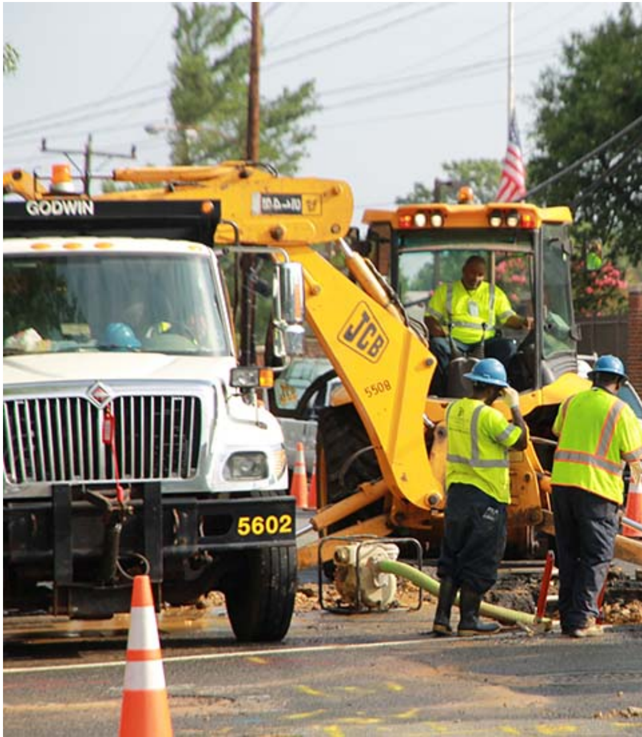
Figure 1: water main repair Copyright © 2018, Gerald Recktenwald. All rights reserved.
