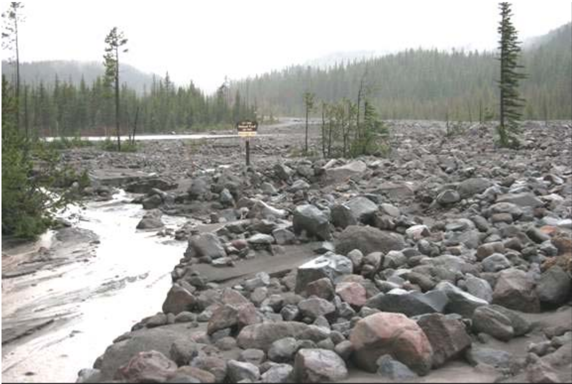
Entrance to White River West Snopark 11/07/2006. Note the little pavement visible in background. This SnoPark will NOT be available this winter!
