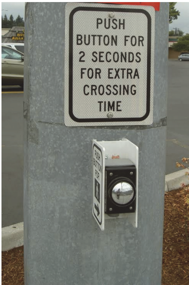
FIGURE 2 Pedestrian phase actuation button (northwest quadrant of intersection of OR-99W and Hall Boulevard, Tigard).
