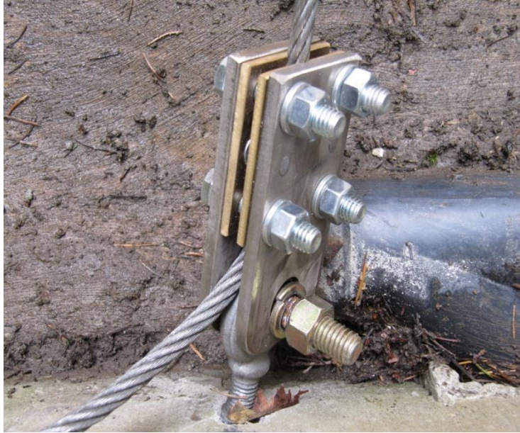
Figure 18: Lower cable clamp and anchor as installed
