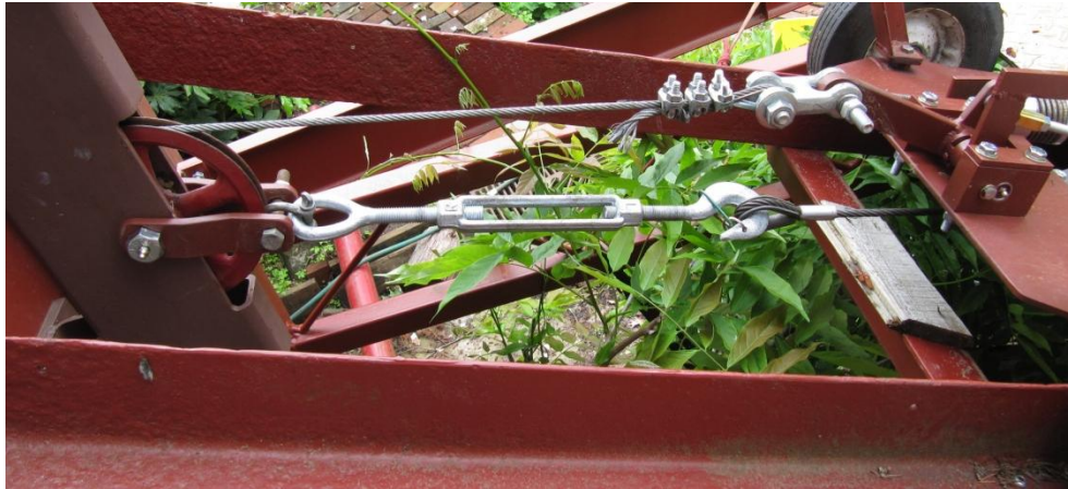
Figure 16: Secondary cable tensioning turn-buckle and pull cable as installed
