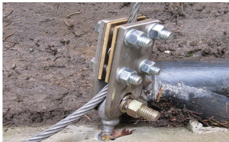
Figure A-10: Lower cable clamp and anchor as installed
