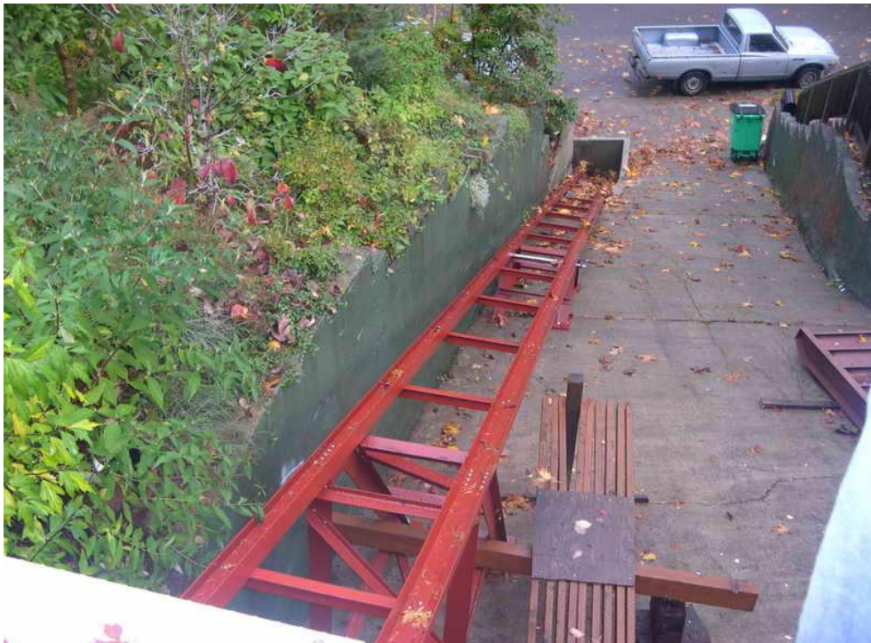
Figure 1: Tramway as viewed from upper landing. Tramway is approximately 77 feet long and descends at a 30 degree slope from the residence to the street.
