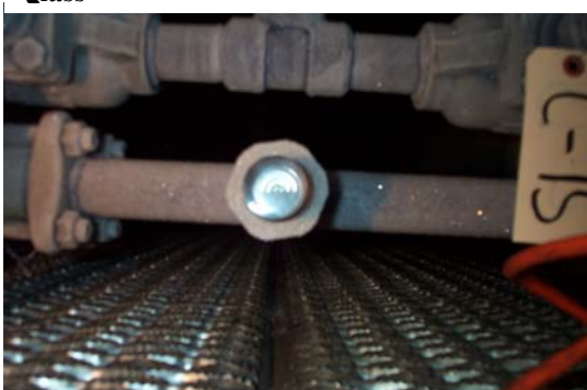
Figure 9-Float drainer exit sight glass
