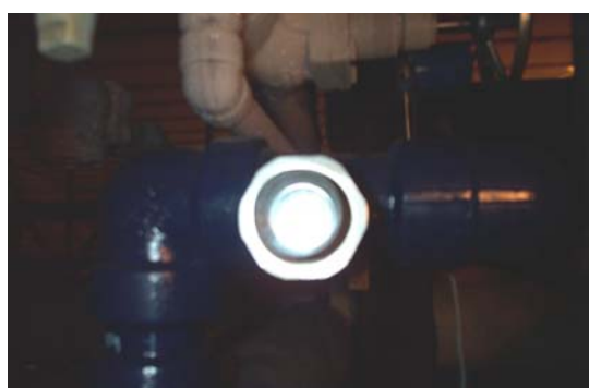
Figure 10-Flow separator gas return sight glass
