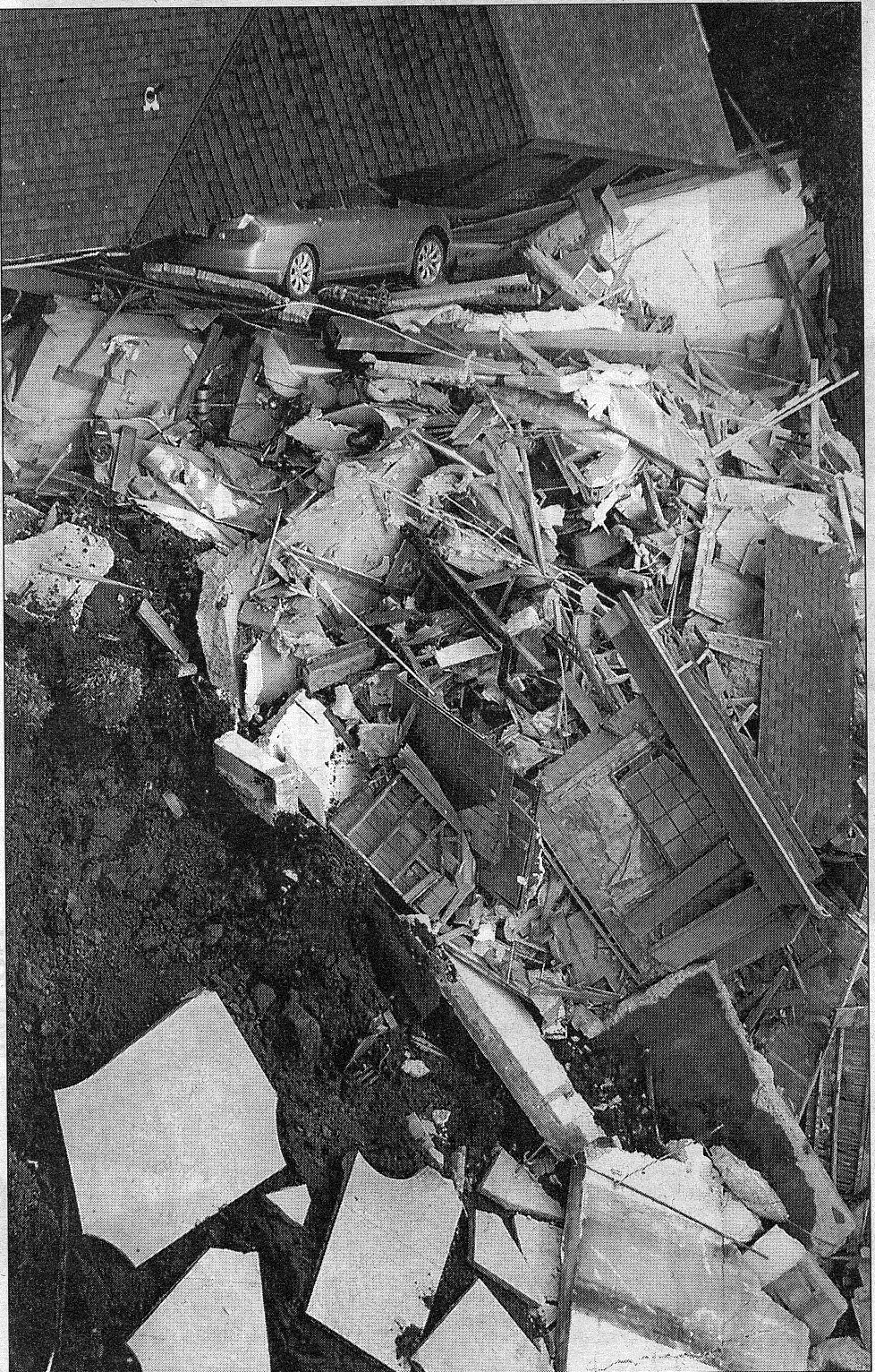
A landslide destroyed a Southwest Portland home and heavily damaged others around it. As the home slipped down the hill, neighbors called 9-1-1. "Your neighbor's house fell down the hill?" a dispatcher asked one neighbor in disbelief.
